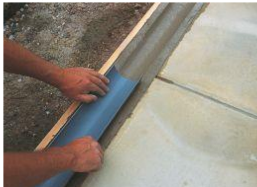
Fig. 5.4: pressing the guttering into wet concrete
