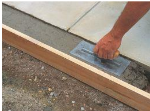
Fig. 5.3: filling the channel with concrete
